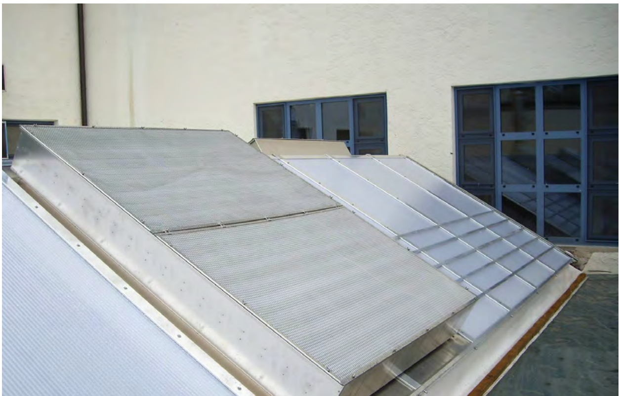
Top view of the roof after renovation
