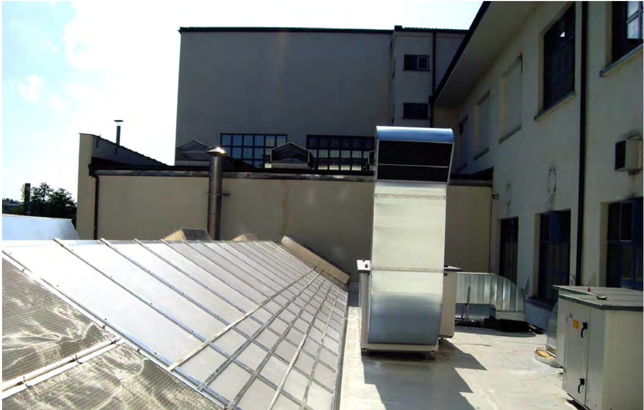
Top view of the roof after renovation
