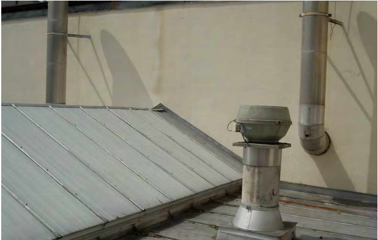
Top view of the roof before renovation
