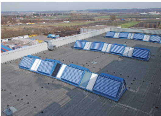
SMOKEJET in a DELTAUGHT polycarbonate roof light by roda as SHE and ventilation unit
