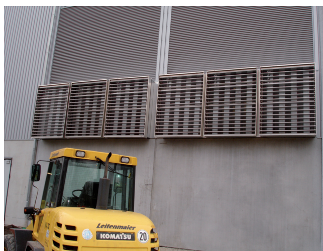
Air-inlet louvre SMOKEJET with splitter-attenuator
