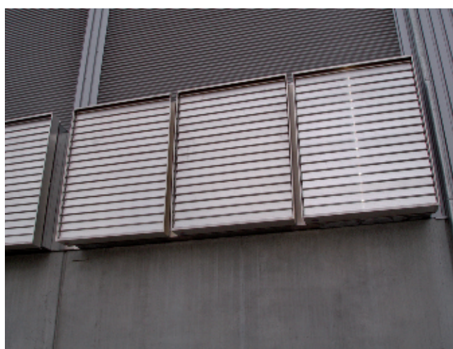
SMOKEJET as an air-inlet louvre
