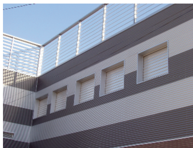
Air-inlet louvre SMOKEJET integrated into a wall construction
