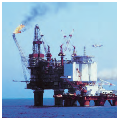
FOGTEC systems on ships and oil platforms
