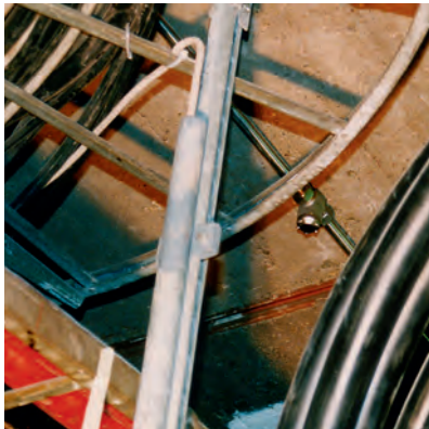
Easy installation of nozzles on the ceiling
