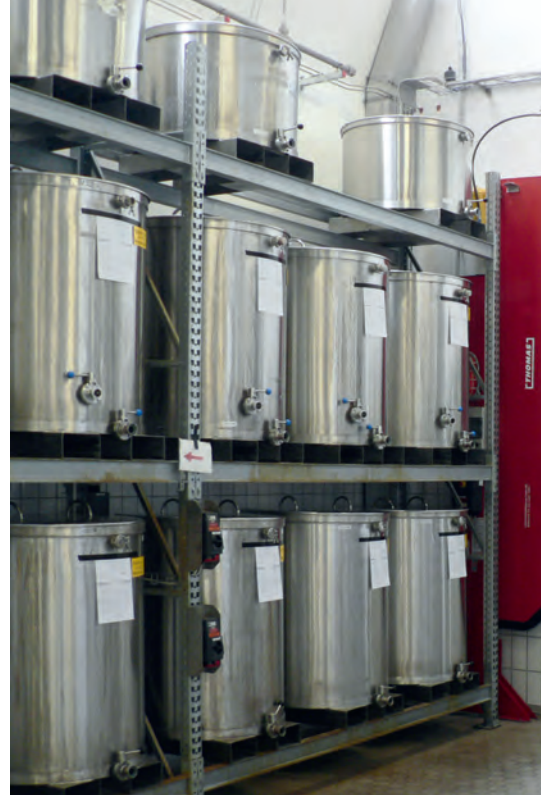
Flammable liquid storage
